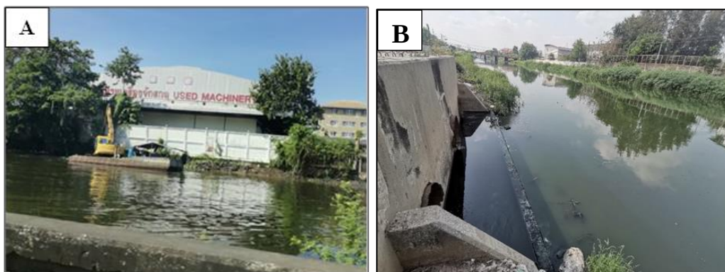
Figure 19: (A) Drainage Cleaning and (B) Drain Outlet without Litter Trap
