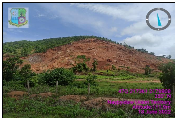
Figure 10. Quartzite Quarry at Wetthoe Mountain region
