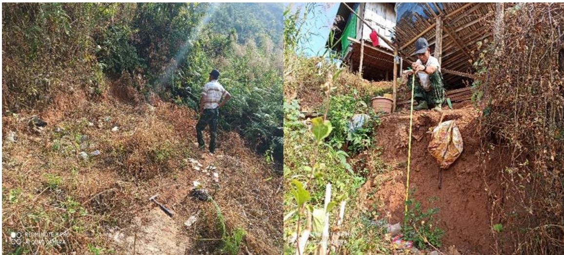
Figure 7. Both tensile crack (left) and step crack (right) in site No.8
