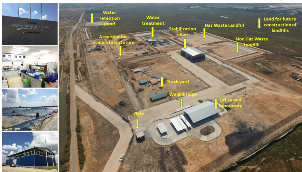
Figure 2: Waste management facilities in Golden Dowa inside Thilawa SEZ
