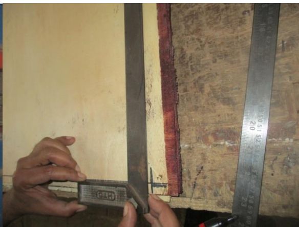
Figure 12 Marking and measuring of plywood
