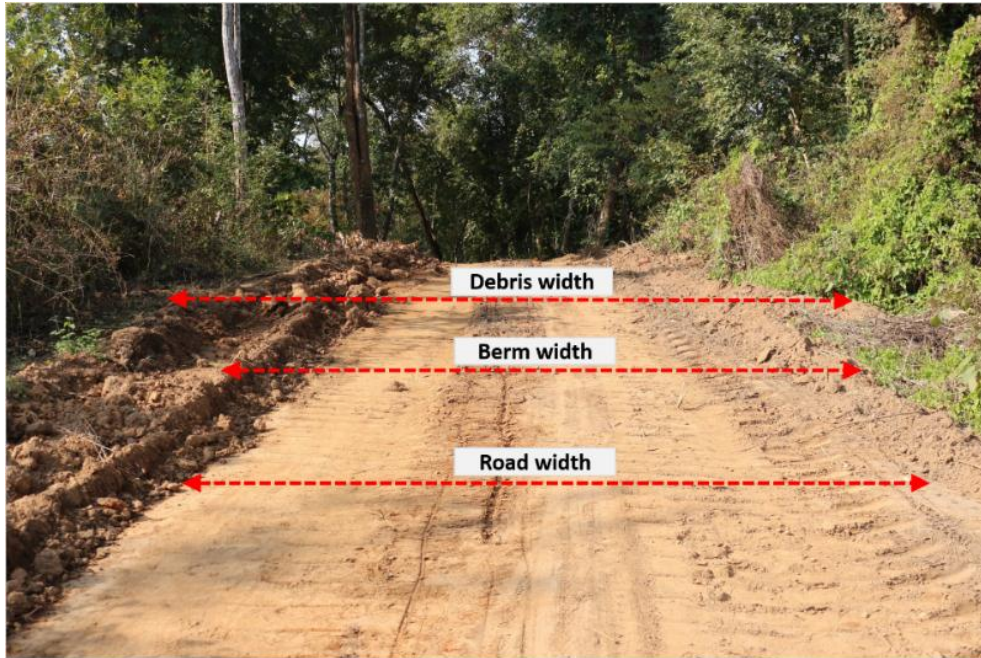
Figure 2. The position for measuring the road width, berm width and debris width.
